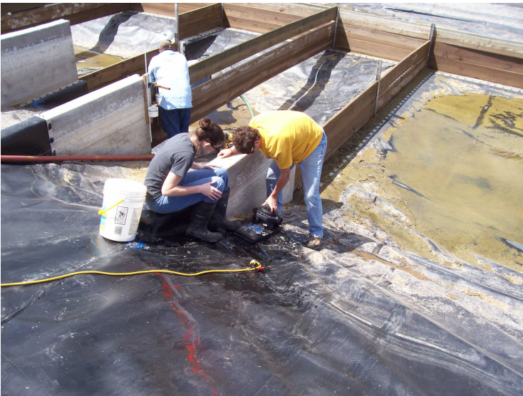
Vacuum box testing
