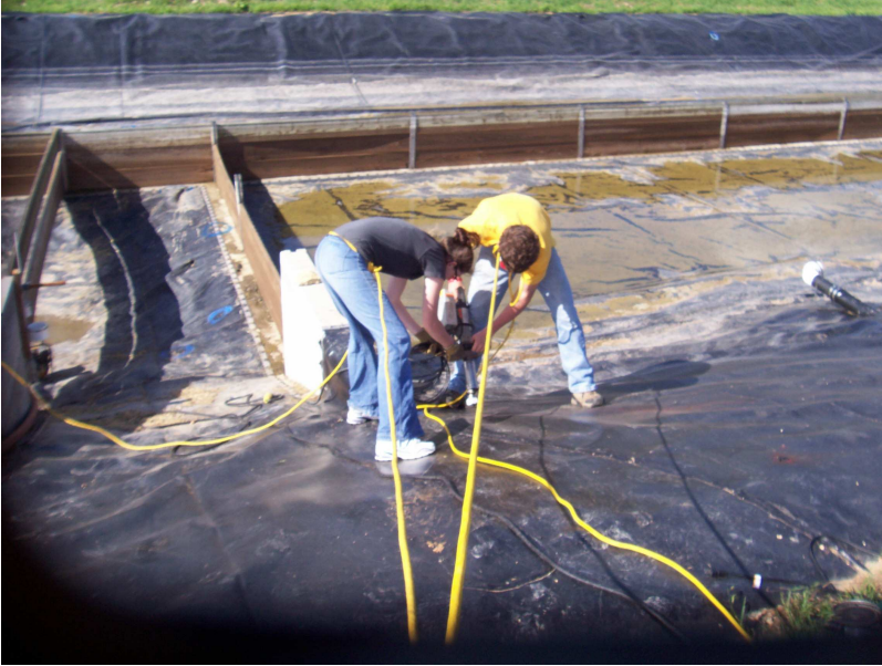
Repairing hole on south side-slope.
