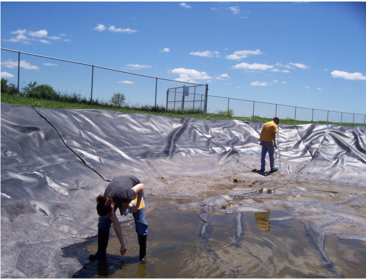
Probe testing for gaps in seams.
