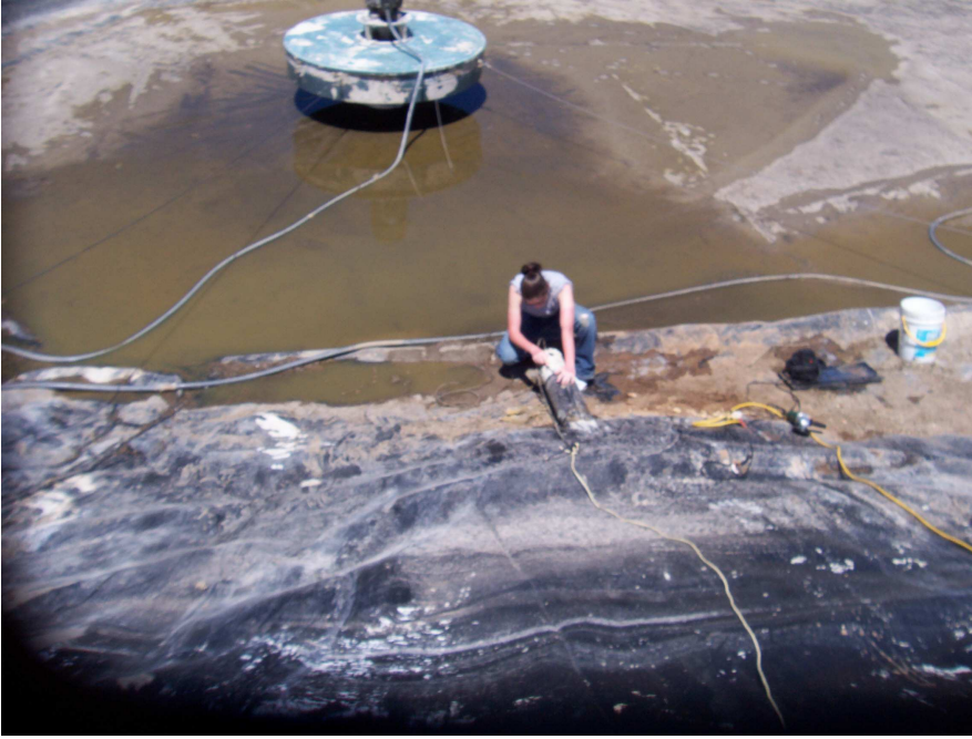
Probe testing steel band attachment of PE skirting to PVC pipe.
