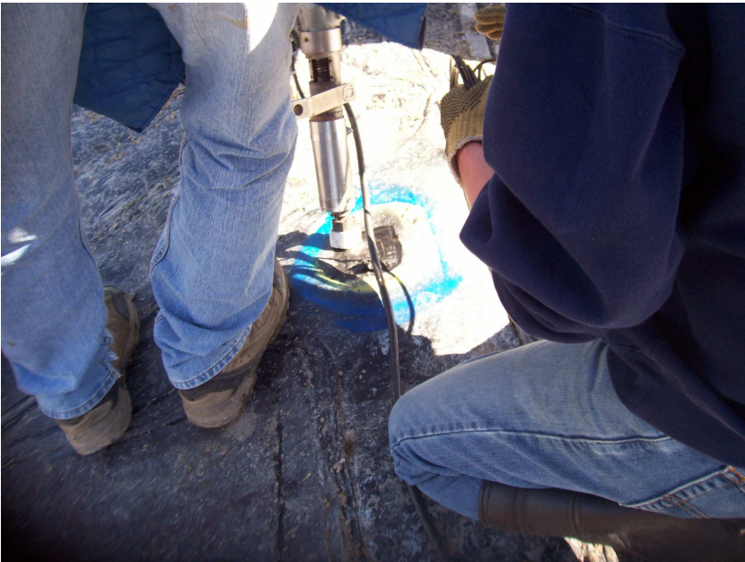
Welding the leaking epoxy glued patch.
