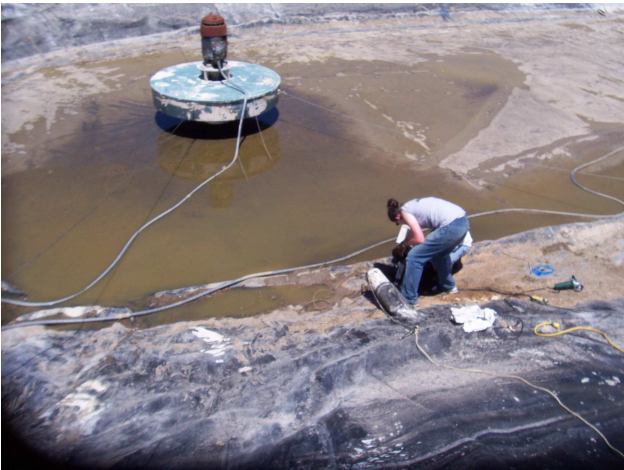
Prepping concrete/Poly-Lock interface with abrasion before sealing with two part epoxy. Note remainder of concrete pad too covered with sludge to inspect well enough.
