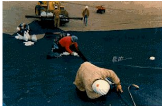
Figure 6 - As it starts to rain, should we wipe the liner dry ahead of the welding to finish a corner panel and ensure the subgrade does not wash? Or should we stop immediately?
