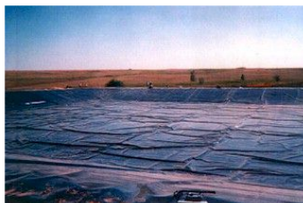
Figure 5a - Retention Pond Liner During Heat of Day Showing Wrinkle Development
